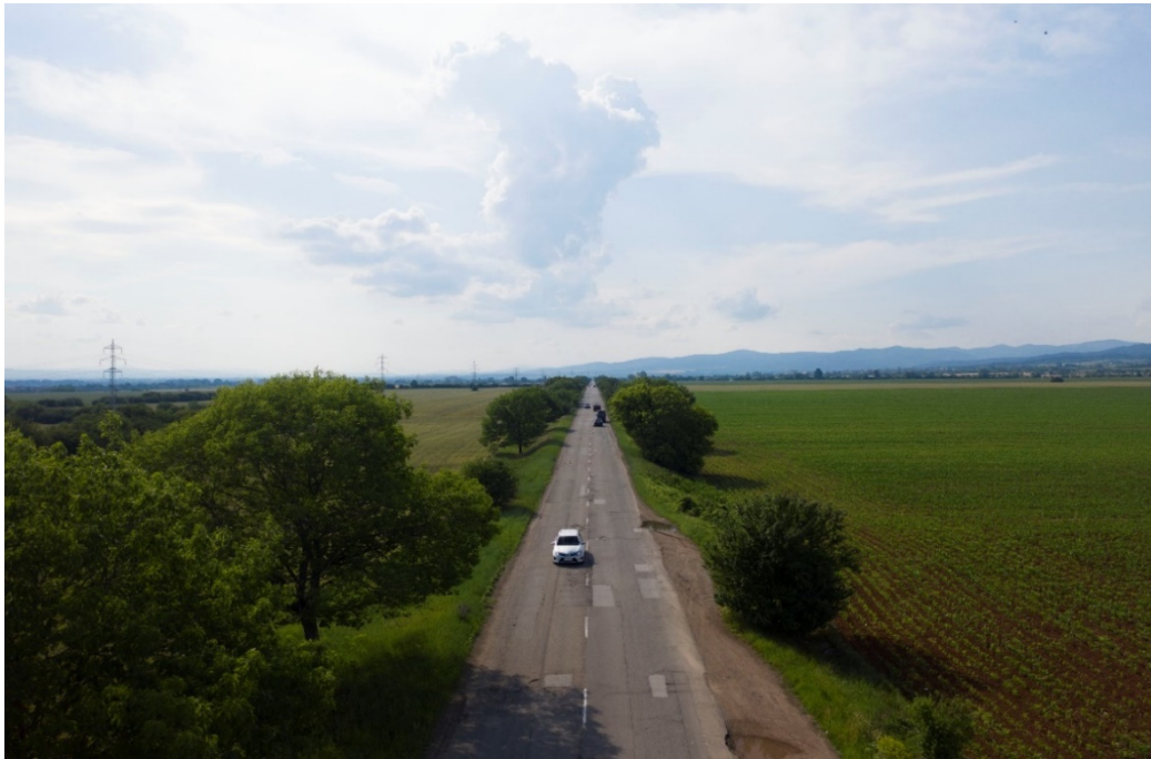
Figure 6. Aerial overview of the roadway used for the study.
