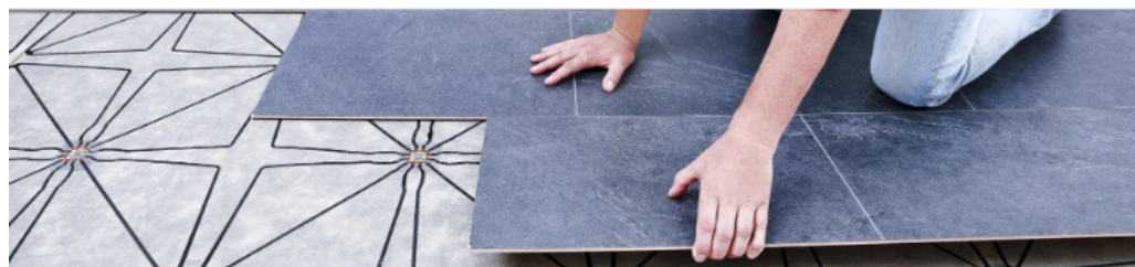
Figure 6. Example of a SensFloor ® use case. To provide additional protection, flooring is positioned above a sensory layer.
