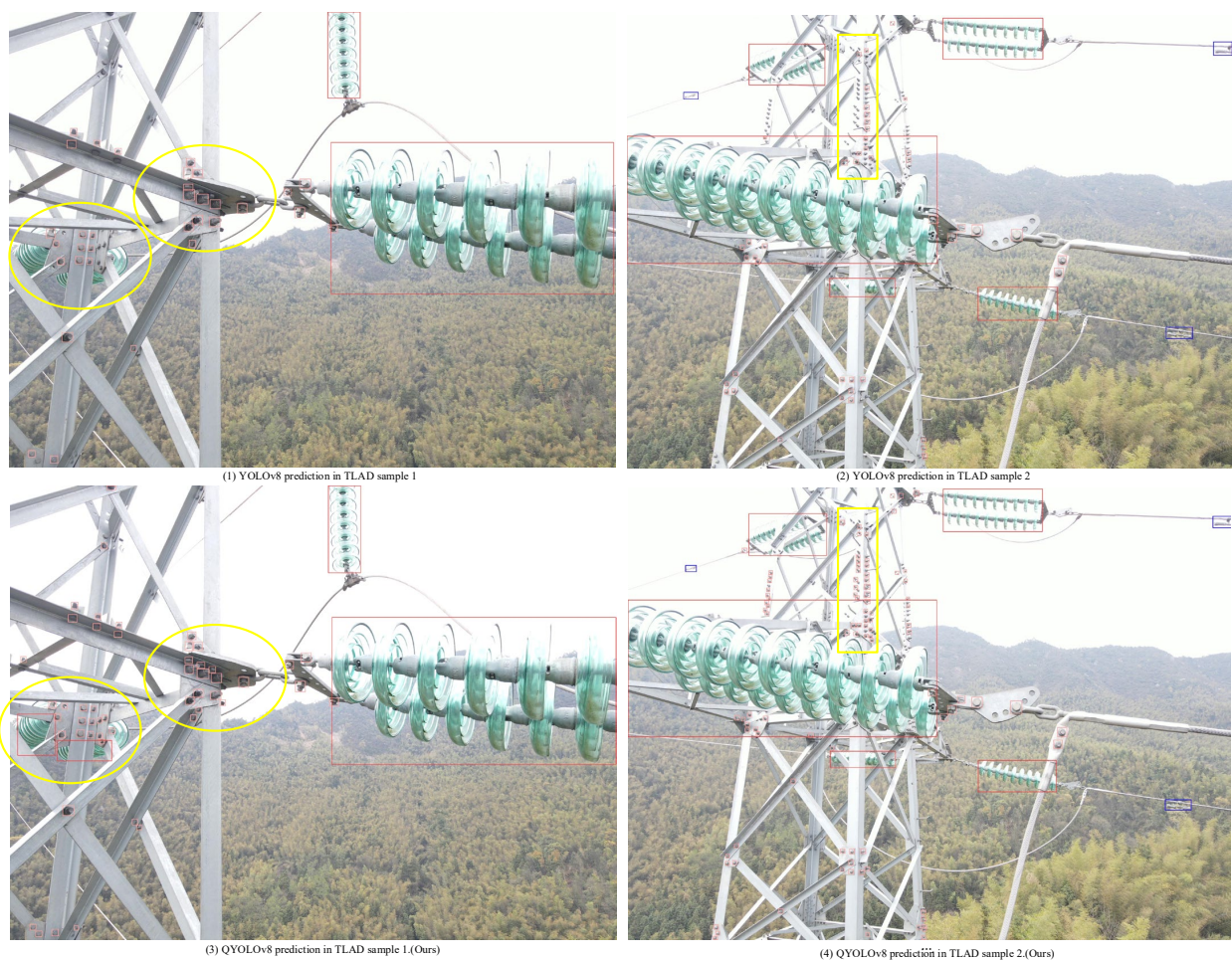
Figure 7. Object detection results based on QYOLO and YOLO. The red boxes indicate the recognized targets as insulators, the pink boxes denote screws, and the blue boxes highlight impact hammers. They emphasize the areas of significant difference that both models need to focus on.
