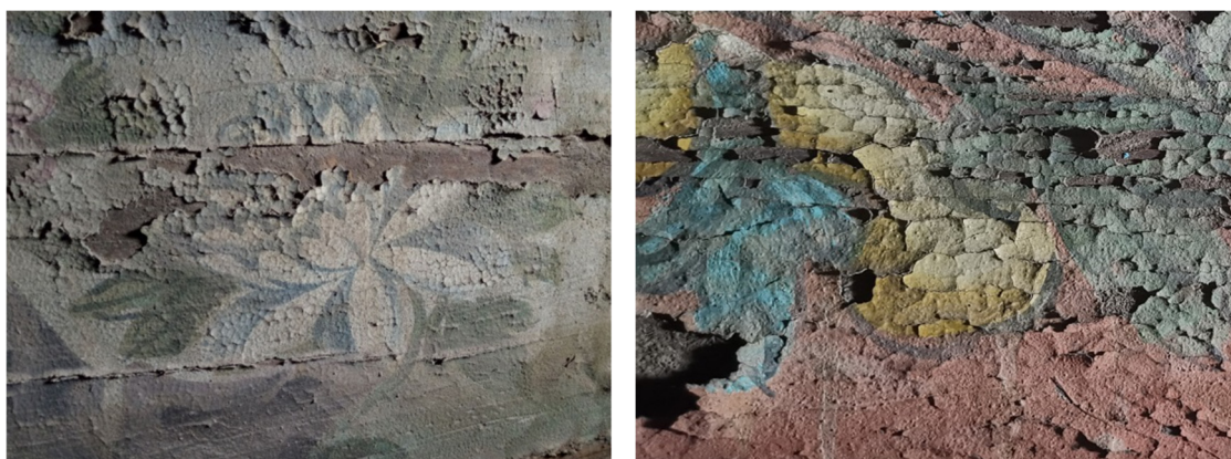
Figure 1. The color painting surface of Sanyou Xuan, the Forbidden City. Due to the synergistic effect of light and salt, the surface of color painting appears powdering, peeling, and warping.
