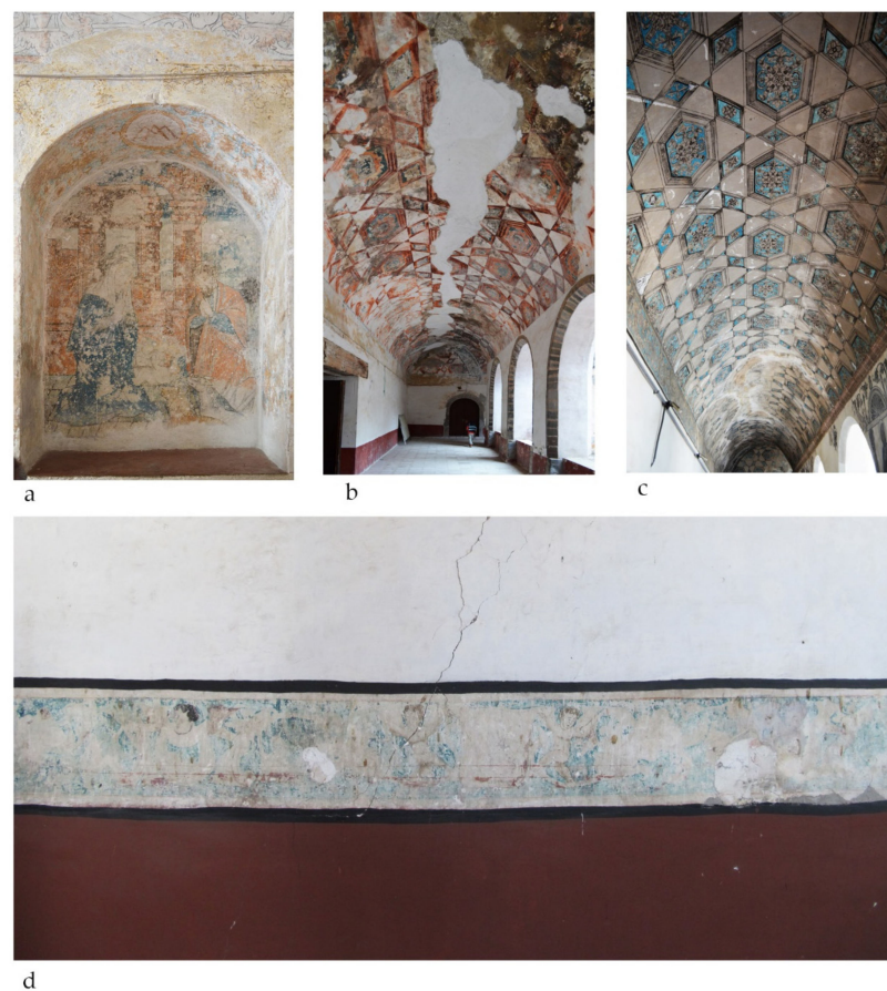
Figure 1. Examples of different hues of blues used in XVI century wall painting. From these wall paintings, very small samples were taken for XRF, SEM-EDS and XRD: (a) Tezontepec, (b) Ocuituco, (c) Oaxtepec, lower cloister and (d) Oaxtepec, upper cloister.
