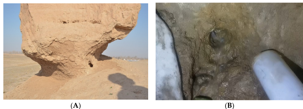
Figure 8. Water deterioration in arid and damp environments. (A) Sapping caused by water transport; (B) water pouring.
