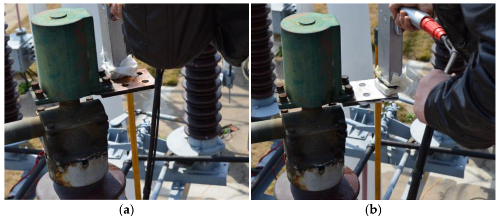
Figure 9. On-site brush plating processing diagram for large instrument parts. (a) brush plating before, (b) brush plating after.
