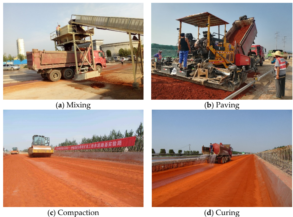
Figure 6. Plant mixing construction of Bayer red mud in a project.
