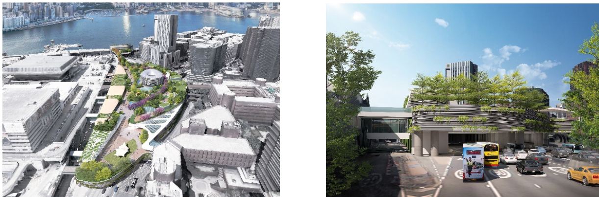
Figure 7. Green Deck Project lead by the Hong Kong Polytechnique University in the Cross-Harbor Tunnel (Kowloon, Hong Kong). This project combines harmonically green roofs and walls with architectural mortar using \text{TiO}_2 and recycled glass for air-purifying purposes [56].
