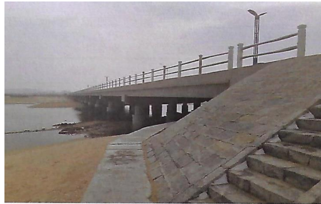
Figure 2. Photograph of the project.
