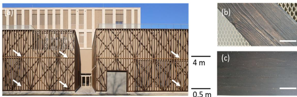
**Figure 1.** Exterior view of the InnoRenew CoE building with designated sampling points marked with arrows at heights of 0.5 and 4 m, strategically distributed to the left, middle, and right positions on the west-facing façade. (a) Close-up photos of the wood facade coated with Biofinish (b,c) Scale bar = 5 cm.
