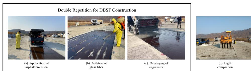
**Figure 1.** Glass fiber-reinforced polymer-modified DBST construction procedure.
