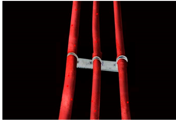
Figure 16. Stitching results for the segment A cable images.
