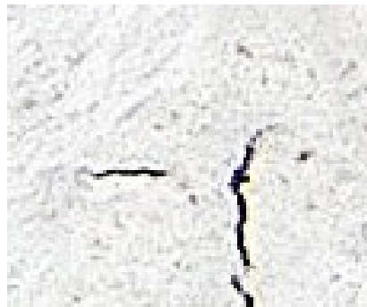
Figure 7. Cracking of the coating due to differential swelling of the wood and coating.
