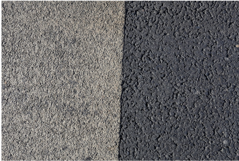
Figure 1. A hot high friction surfacing (HFS) coating applied to a 10 mm Thin Surface Course System.
