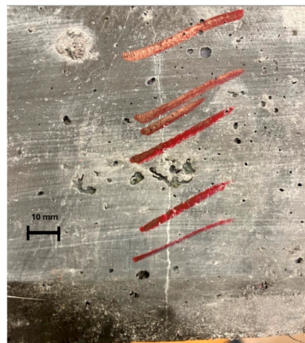
Figure 12. Formation of calcite immediately after the cracking load of 28 days (S0.3 with water curing).
