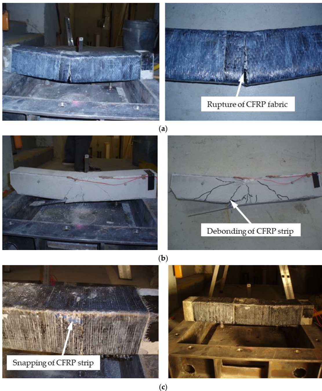
Figure 8. Failure modes and cracks pattern during a 1 m drop weight impact test of RC beams of (a) B2, (b) B3, (c) B4.
