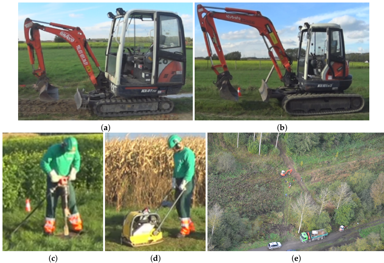
Figure 4. Database machines: (a) big excavator; (b) small excavator; (c) pneumatic hammer; (d) plate compactor; and (e) aerial view (figures (a–d) are reproduced with permission from [30]).
