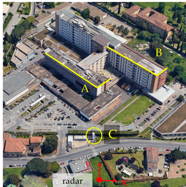
Figure 10. Aerial view of the illuminated area. The radar position is highlighted by the red dot. The main targets present in the scene are highlighted in yellow. A is the upper edge of the closest building, B is the upper edge of the farthest building on the right, C is a metallic tank with industrial gas.
