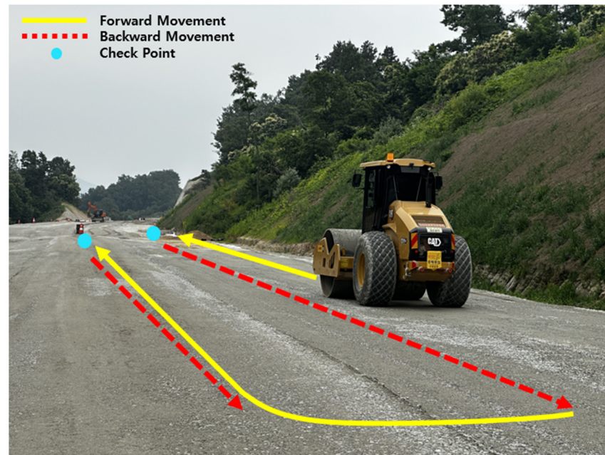
Figure 2. General movement of roller at construction site.
