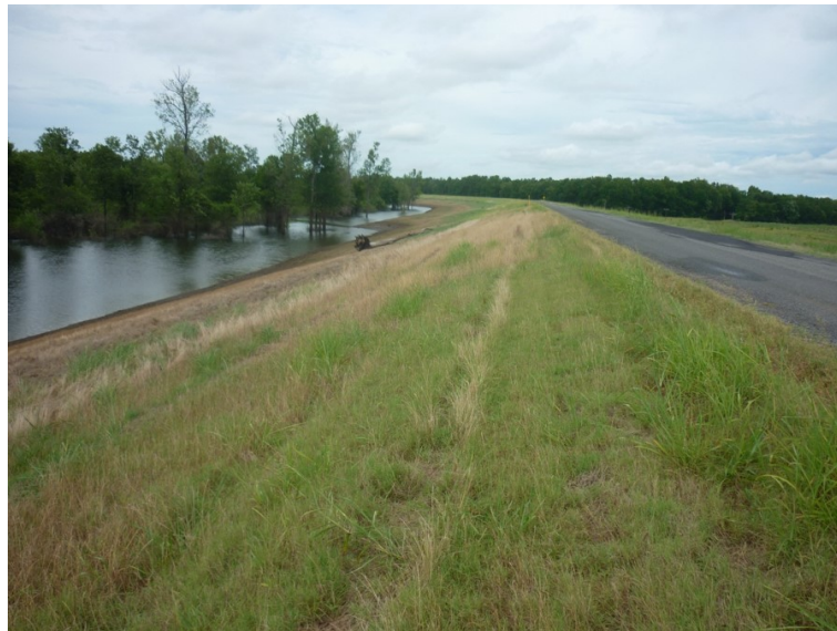
Figure 4. Earthen Levee on the banks of Albemarle Lake, MS, USA, a Mississippi River oxbow.
