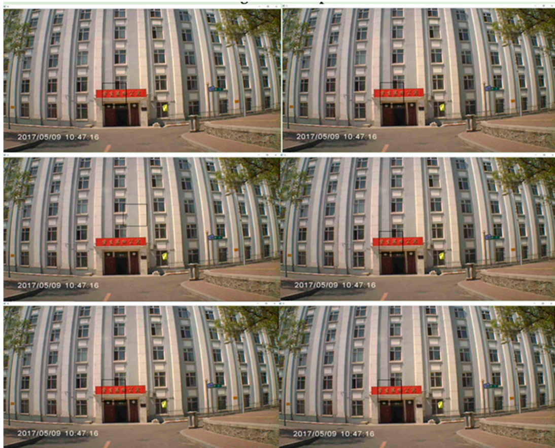
Figure 10. Six matching techniques at time 10:47:16.
