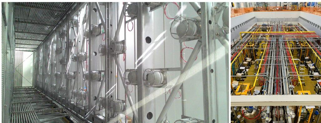
**Figure 13.** (Left): Deployment the upgraded ICARUS-T600 PMT system behind a wire plane of one of the four TPCs during the overhauling activities at CERN. (Right): Status of the ICARUS-T600 plant at Fermilab before the beginning of the cryogenic commissioning in 2020.
