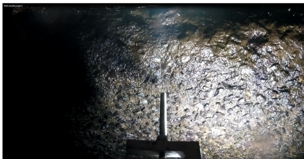
(a) Photo of concrete sewer.
