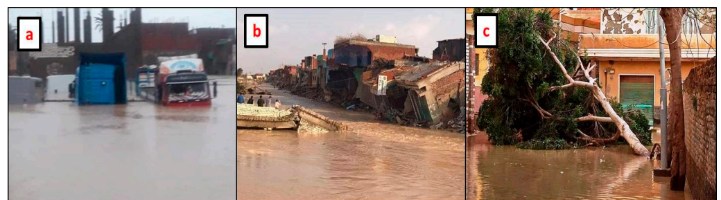
Figure 10. Field photographs showing the destructive impacts along the intersection of the outlet of the Wadi Al Rishrash catchment at the Al Dismi village after the flood event of 13 March 2020, including damage of vehicles (a) drowning of urban centres (b), and damage of trees (c). The location of the Al Dismi village is highlighted in Figure 1.
