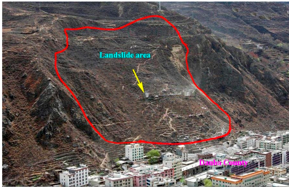
Figure 2. The scope of the Danba landslide.
