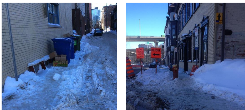
Figure 4. Examples of barriers on the sidewalk.
