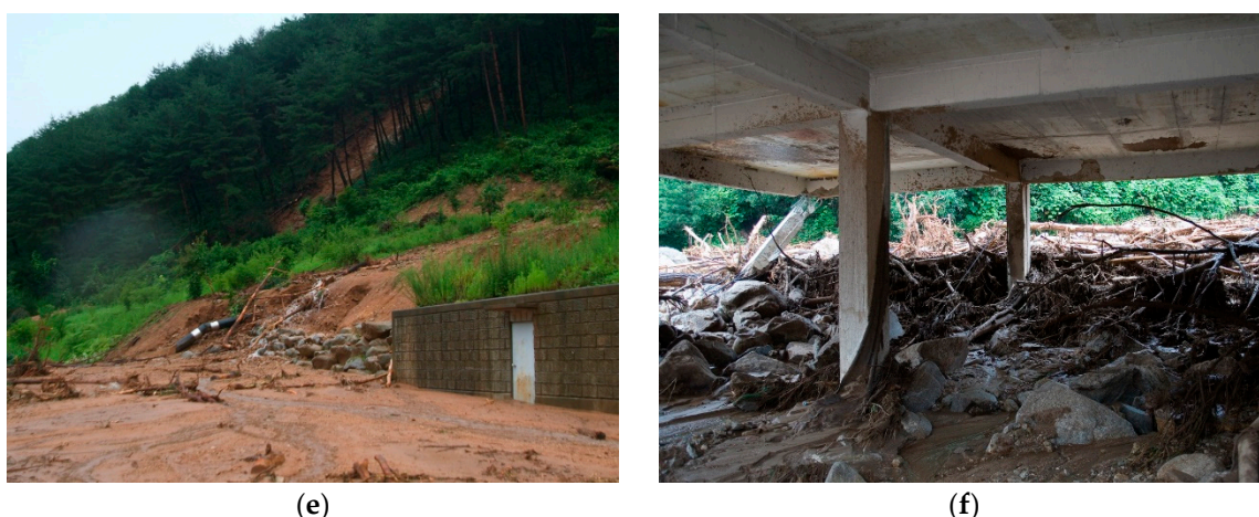
Figure 3. (a)–(e): observed landslides and (f) debris deposit.
