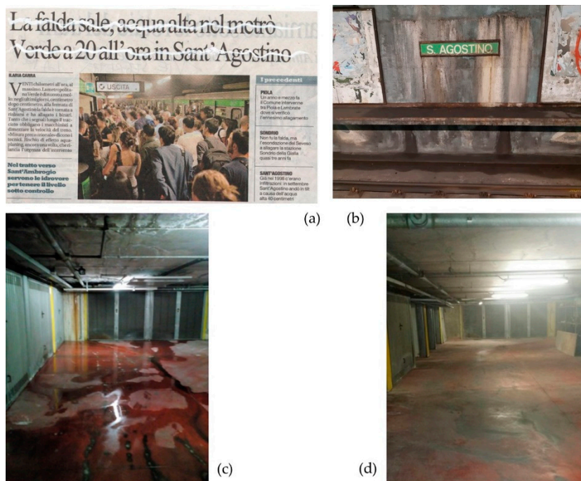
Figure 12. (a) Newspaper article of “La Repubblica” (2 July 2013), dealing with flooding episodes in Sant’Agostino station. (b) Flooding evidence in Sant’Agostino station (8 September 2020). (Image credits to the authors). (c) Flooding evidence in Numa Pompilio public car park. (d) Absence of flooding evidence after waterproofing works in Numa Pompilio public car park. (c,d): images were provided by Rete Irene.
