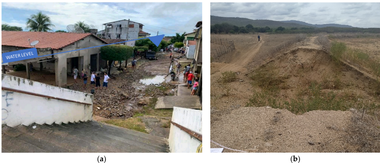
Figure 7. (a) Water level reached during the flood event marked at the walls affected by the flood. (b) Dam breach in a small reservoir upstream of the city.
