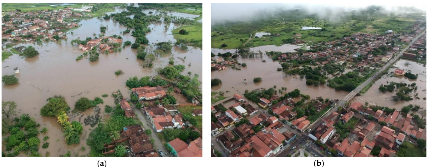
Figure 5. Aerial image of the flood that occurred in March 2020. (a) Downstream of the bridge, a neighborhood isolated by the river. (b) Aerial view of the city bridge failed to drain the entire volume of water—one part was accumulated on the upstream side.
