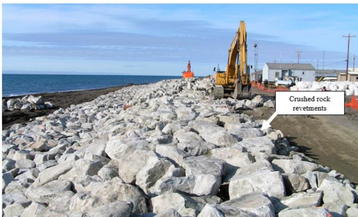
Figure 8. Rock revetments along the Alaskan Arctic coast adapted from [75].
