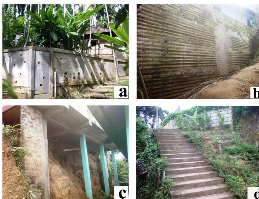
Figure 6. Construction of protection wall surrounding the (a) houses and (b) locality; changing design and patterns of (c) houses and (d) staircases.
