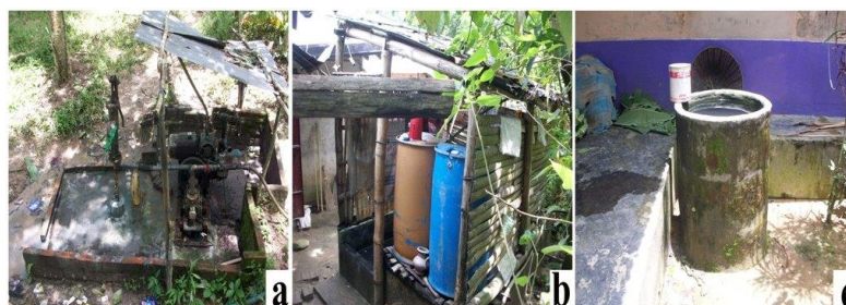
Figure 4. (a) Setting water pump; storing water in (b) plastic drum and (c) cemented rings.
