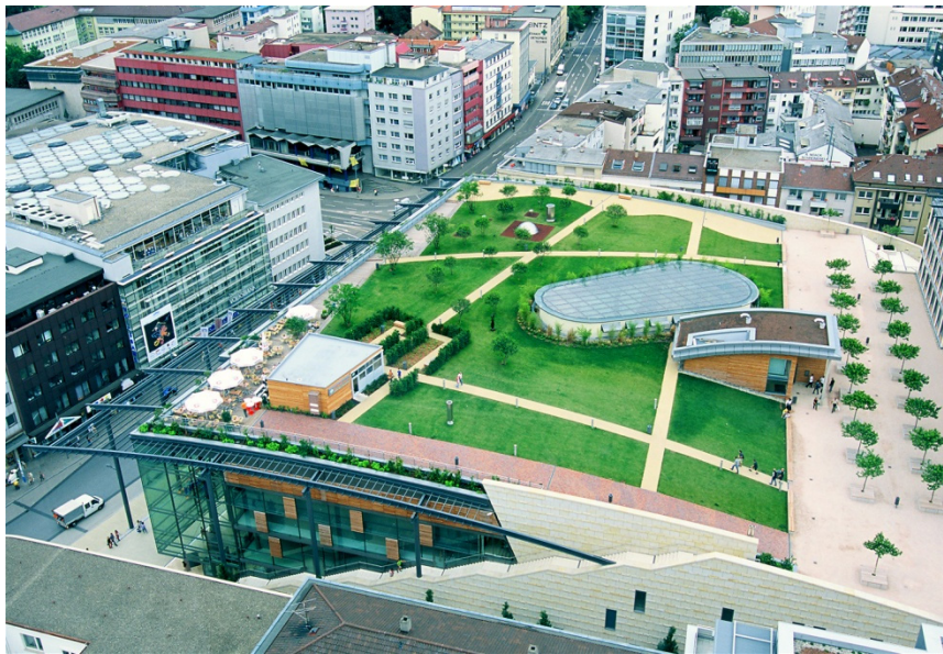
Figure 4. Germany's green roofs.
