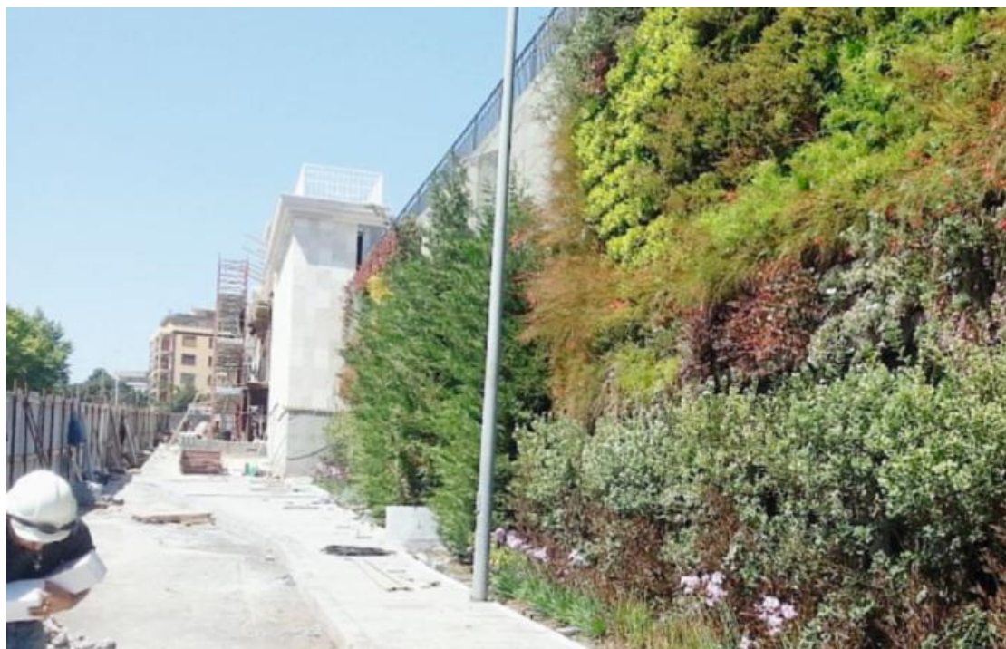
Figure 11. Tondo Gioeni (today, after the realization of the vertical wall).
