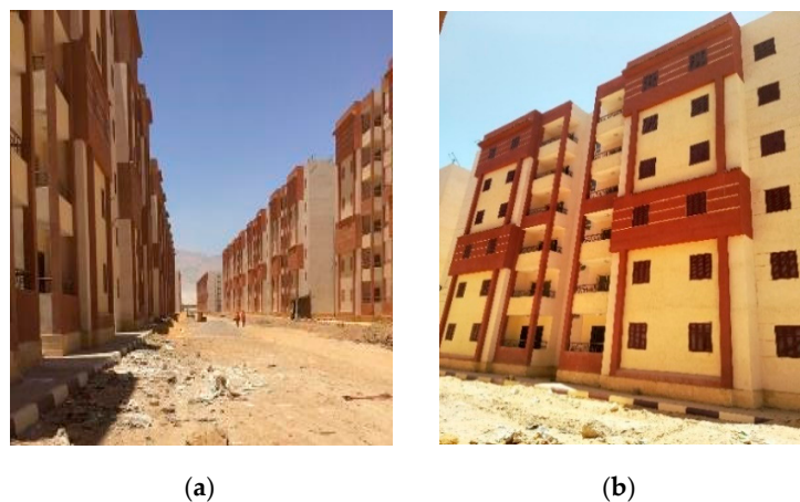
Figure 2. Pictures from the project site; (a) A picture showing the scale of the project; (b) A picture showing the East façade of a typical building.
