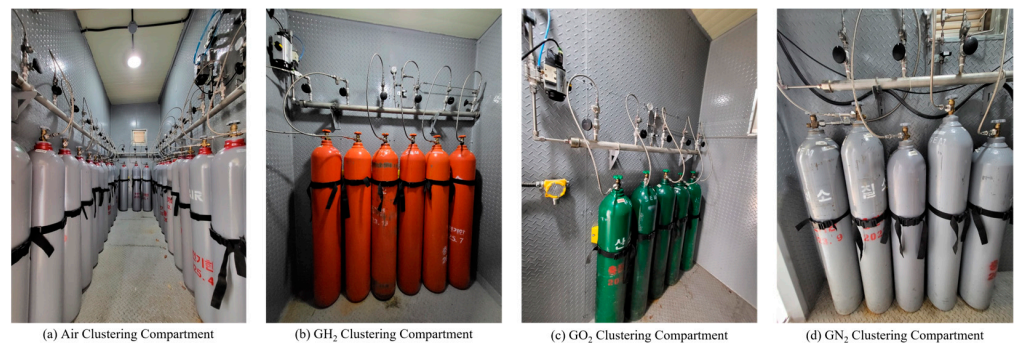
Figure 8. External (a) air, (b) \text{GH}_2 , (c) \text{GO}_2 , and (d) \text{GN}_2 clustering compartments.
