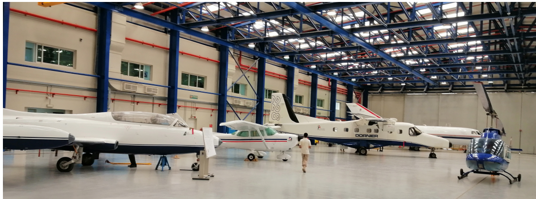
Figure 5. Abu Dhabi Polytechnic Aircraft Hangar.
