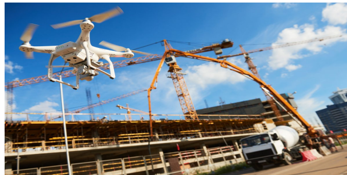
Figure 13. UAVs in construction industry [109].
