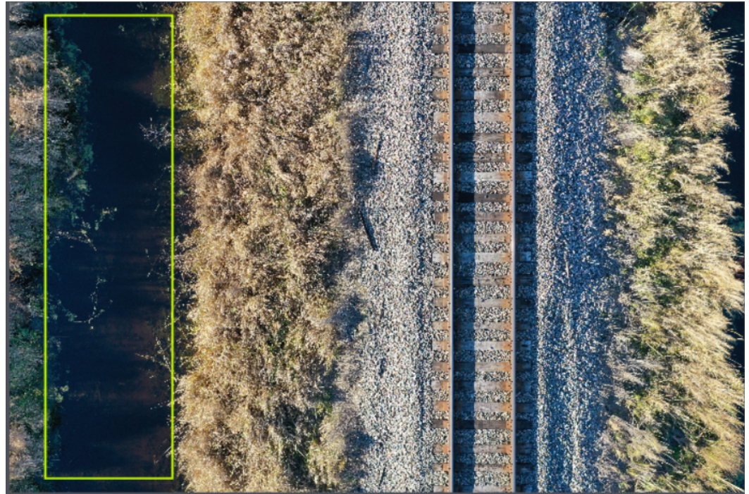
Figure 9. Example of water pooling.
