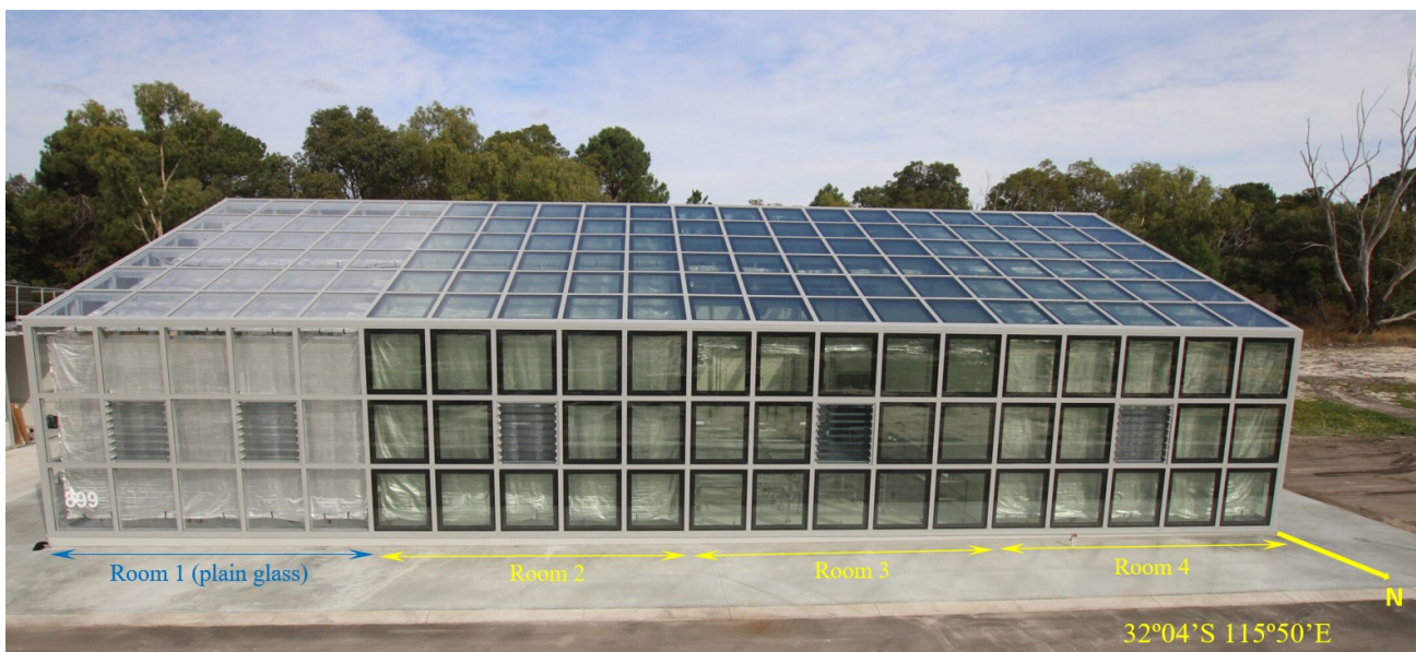
Figure 1. Murdoch University solar greenhouse after its construction and fit-out were completed in Perth (Western Australia) in April 2021. The internal grow-room boundaries are marked; the direction to geographic north and the greenhouse location coordinates are also shown.
