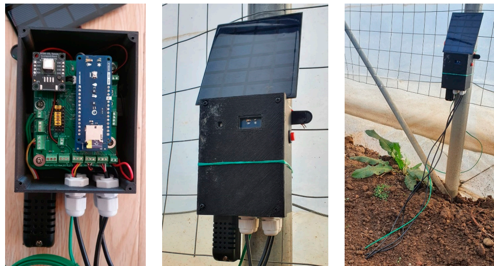
Figure 7. The final wireless sensor node installed in the greenhouse.
