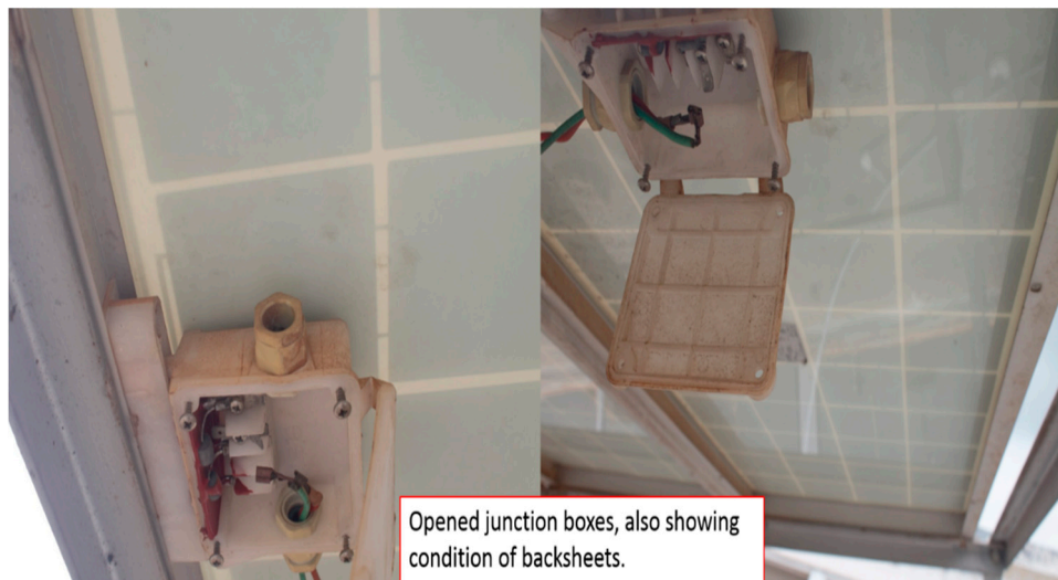
Figure 9. Junction box of modules, also showing backsheet.
