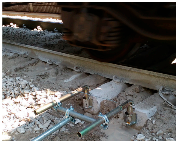
Figure 7. Measurements of the displacement of sleepers using inductive displacement sensors.
