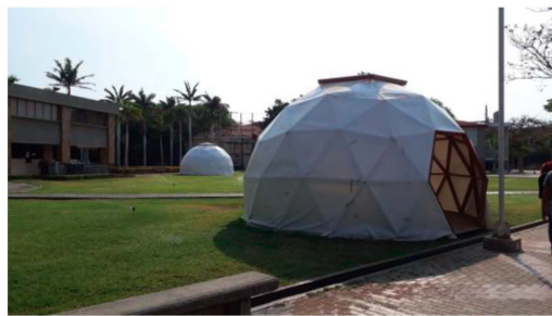
(c) Situation an external view of the dome built.
