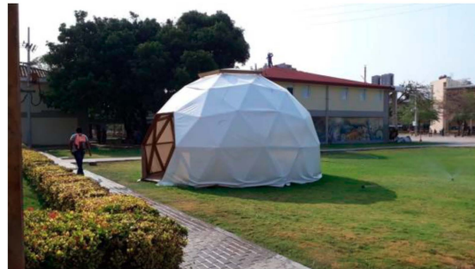
(b) Construction of the internal structure.
