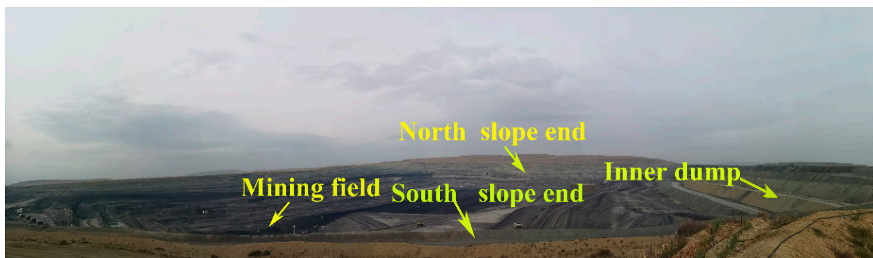
Figure 2. High slopes of Shengli #1 open-pit mine.
