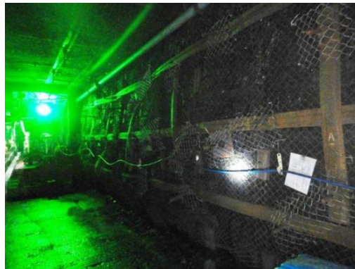
Figure 16. Field observation of roadway stability.
