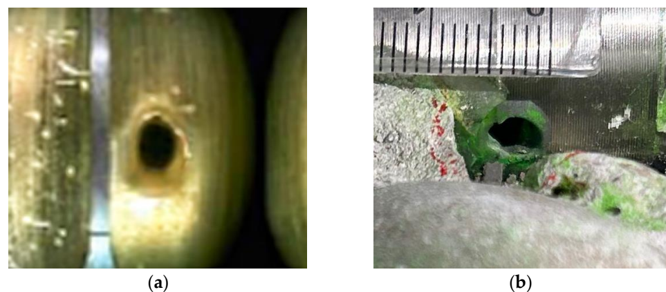
Figure 5. Perforation hole morphology. (a) The perforation hole took place underground in the field, showing an irregular circular hole; (b) the perforation hole made by the new water jetting apparatus, showing a similar morphology with the hole on site.
