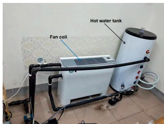
Figure 3. Fan coil and hot water tank.
