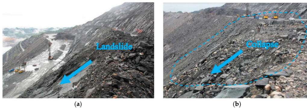
Figure 1. Landslides and collapses caused by rainfall. (a) local landslide; and (b) overall collapse
