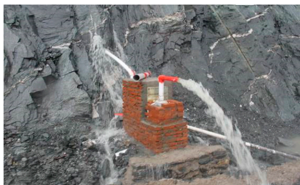
Figure 11. Pipe draining of rainwater and groundwater away from Nanfen open-pit mine slope.
