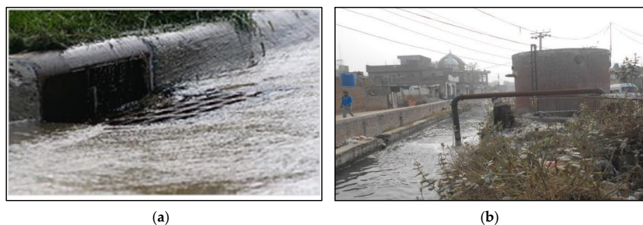
Figure 1. (a) Urban runoff flowing into the sewer drain; (b) sewage outfall into the Charar drain
