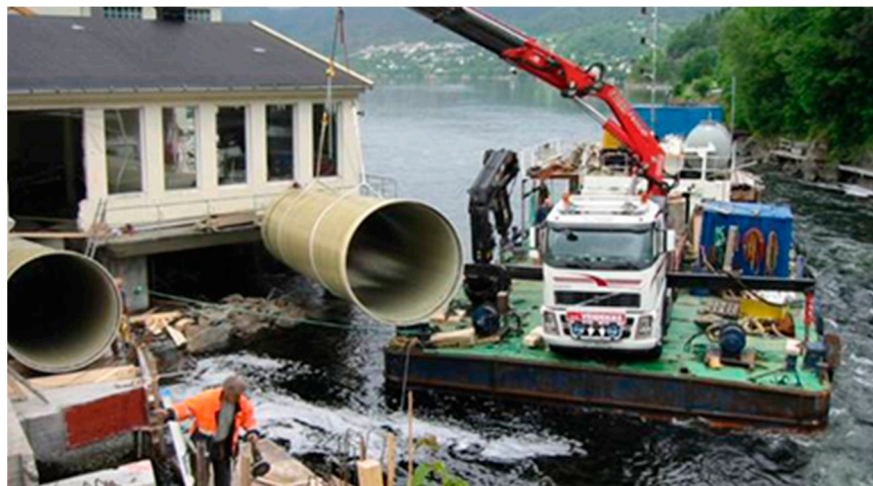
Figure 14. Installation of pipes from barge [18].
