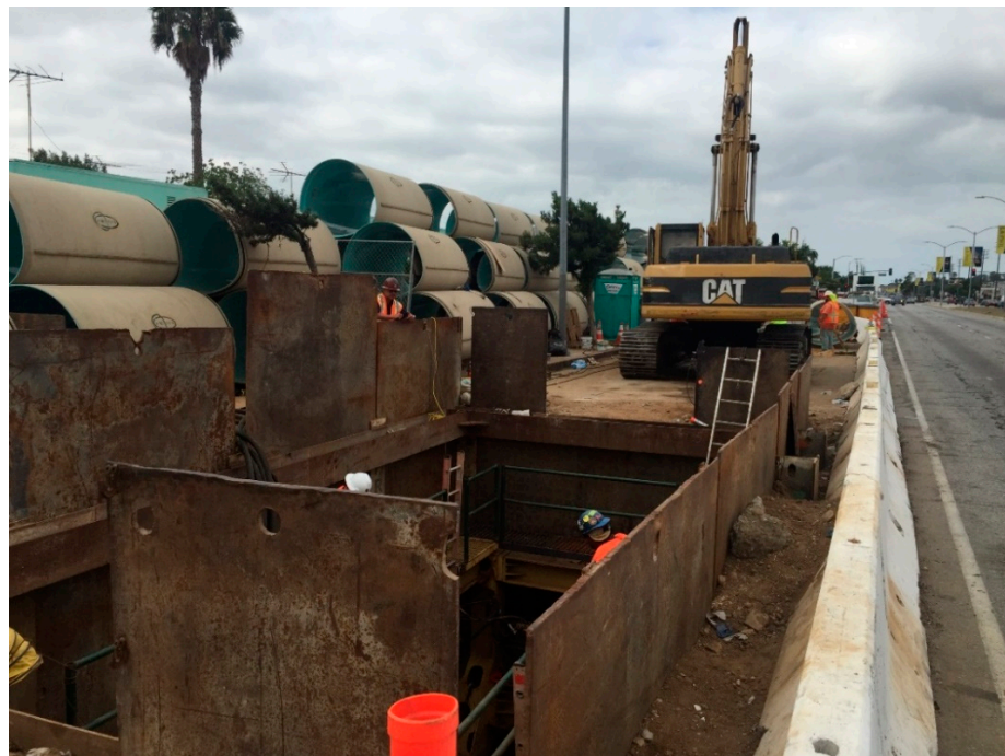
Figure 16. Installation access pit with stored segments of non-circular pipeline [34].
