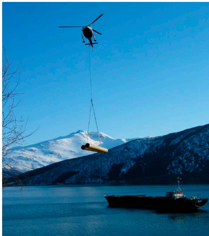
Figure 12. Unloading of pipes by helicopter [18].
