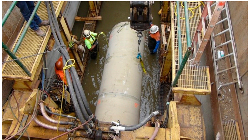
Figure 19. Installation of the segment into the host pipe [34].
